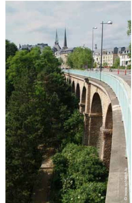
Luxembourg City, “La Passerelle” bridge
